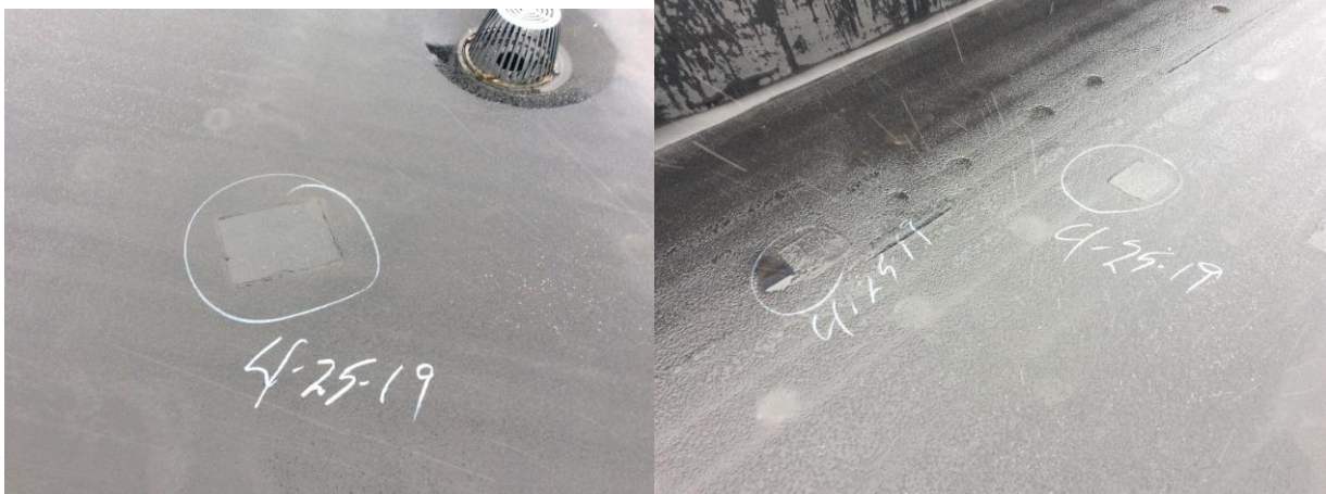
Shows roofing repairs that are dated accordingly.
