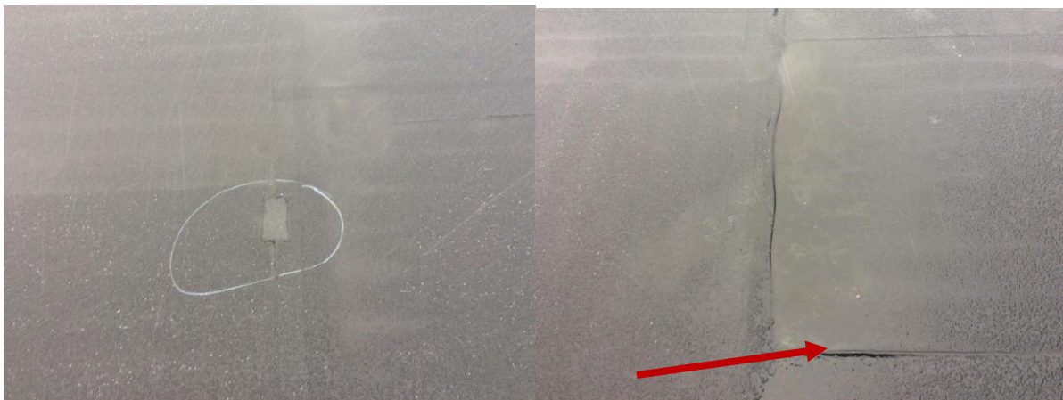
Shows roof repairs and also shows lifting rubber seams.
