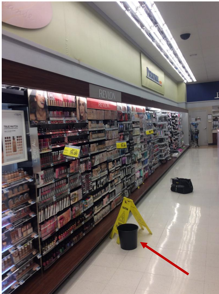
Shows roof leaking on east side of the store active
