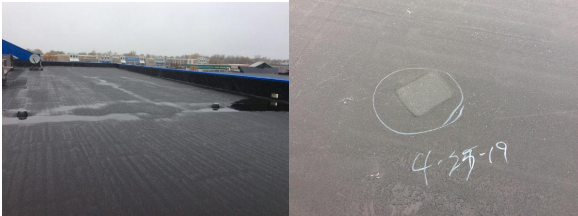
Shows roofing repairs that are dated accordingly.
