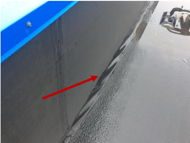
Evidence of failing roof membrane at base of parapet walls.
