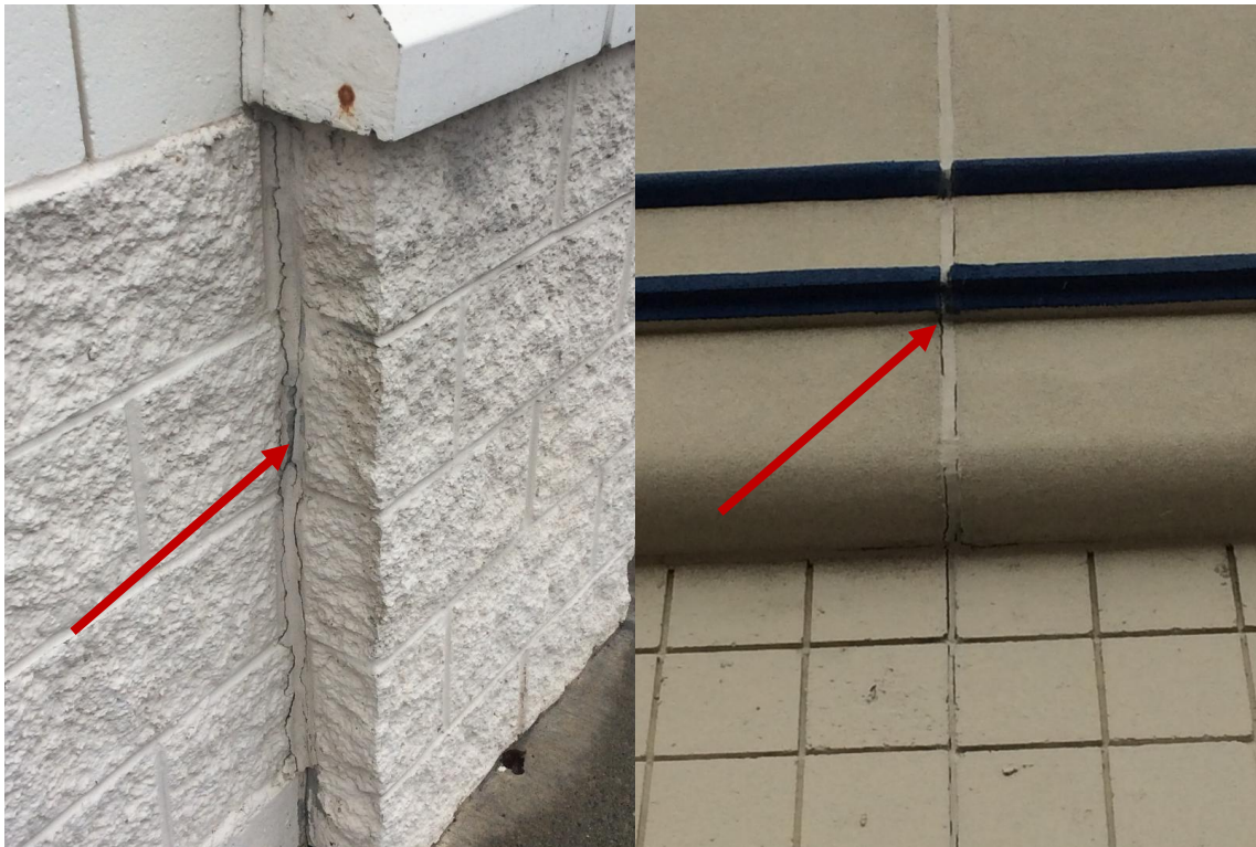
Shows open and failing calking joints that are in need of repairs.
