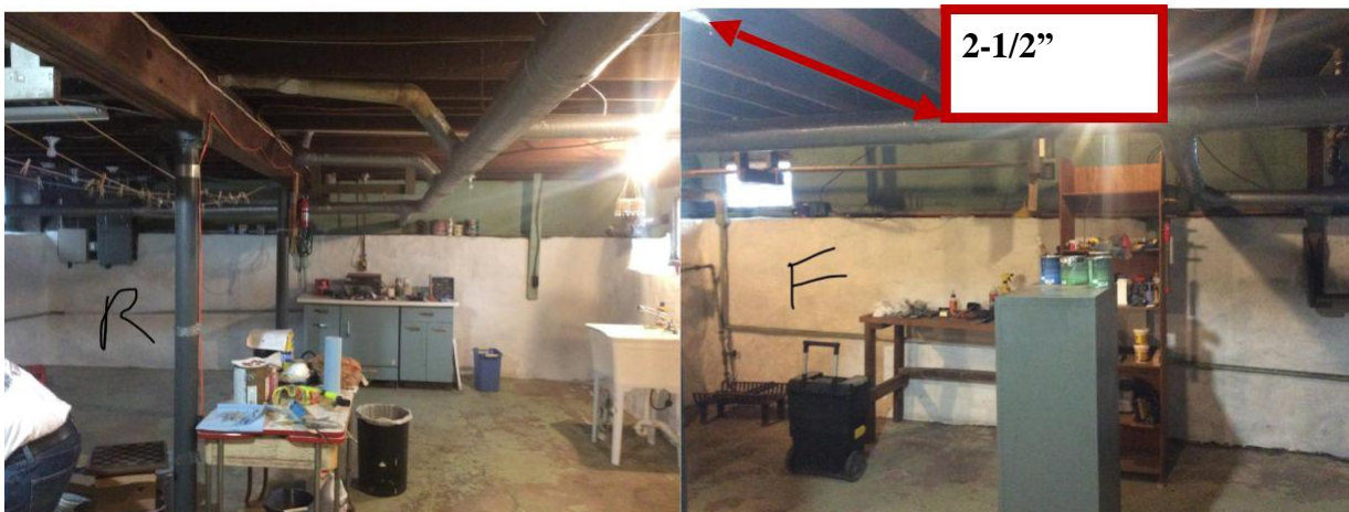
Shows rear and front walls for reference. Note front wall is lower than main wood support beam by 2-1/2".
