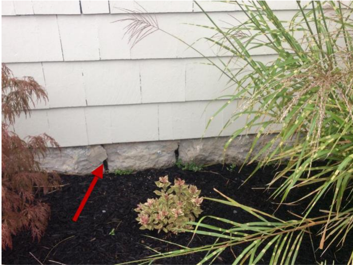
Shows open stone mortar joints at front crawl space wall, mortar any open joints.
