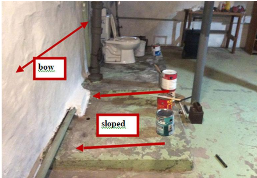
Shows bowing of south wall and slab concrete pad sloped towards wall from settlement.
