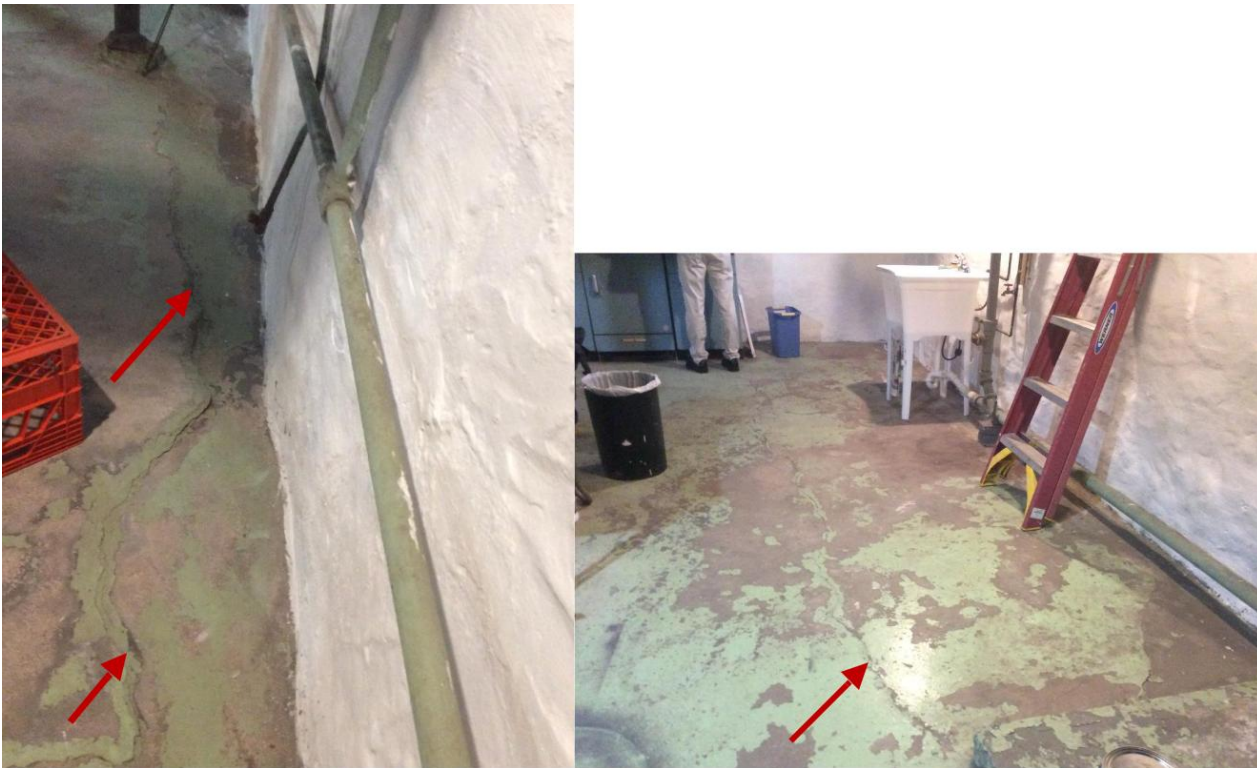
Shows cracked concrete floor along walls indications of wall settlement.
