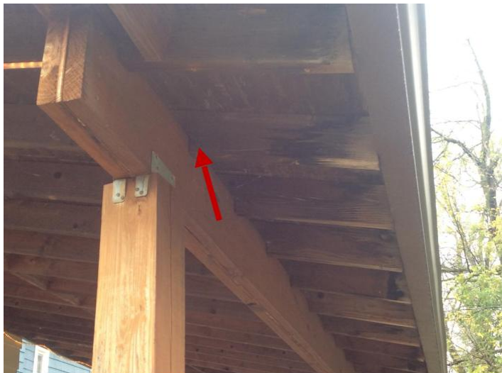
Suggest adding metal tie down straps to secure roof rafters to wood header.
