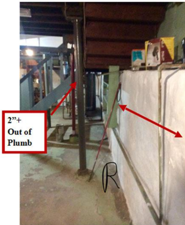
Shows bowing of south wall and slab concrete pad sloped towards wall from settlement.
